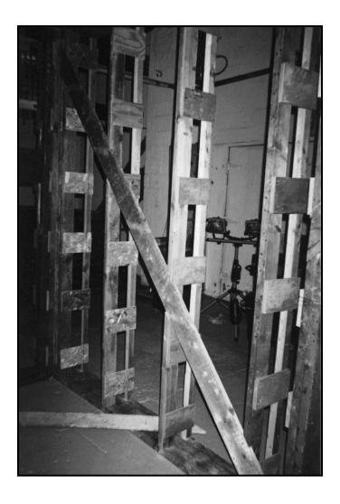
Figure G-1. Larsen energy wall systems constructed by REEHouse
