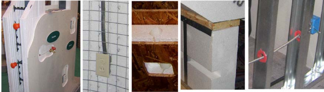
From left to right: Insulated concrete forms with utilities run through spaces routed out of the Styrofoam, insulated spray-on concrete form with conduit run before spraying, SIPS with factory created conduit in insulation, new SIPS with factory created raceway, and steel framing with plastic bushings. Photos from International Builders Show.
