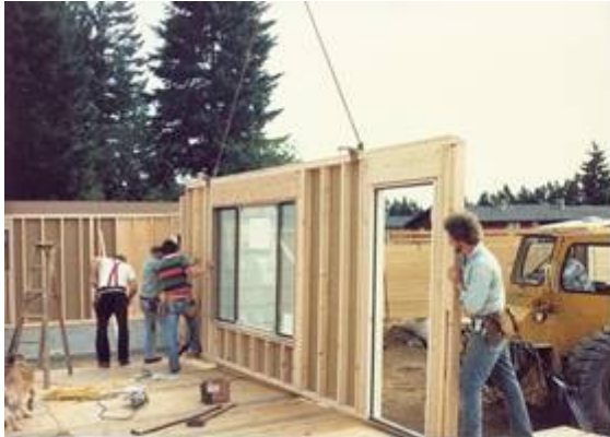
Figure 13: Panelized Building during Construction
