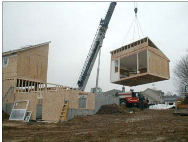
Figure 14: Modular Housing under Construction
