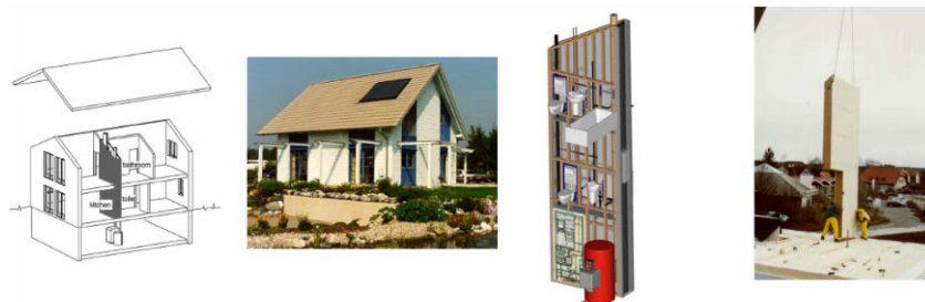
Figure 24: Integrated Multi-Story Utility Wall Prototype 38
