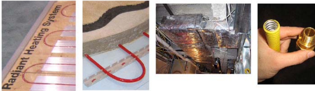
From left to right: PEX radiant heating embedded in sub floor, PEX radiant heating embedded in concrete, traditional ductwork for forced air heating, and flexible gas pipe and a fitting. Photos from International Builders Show.
