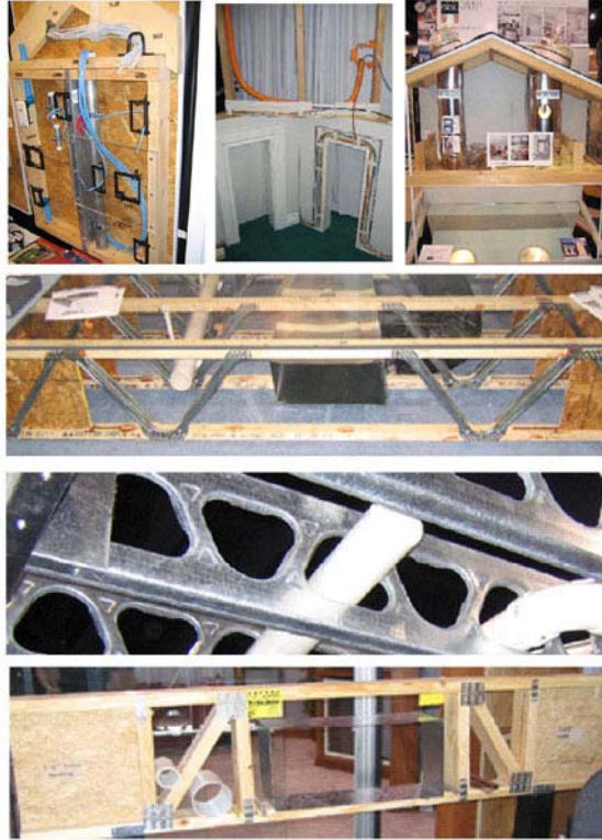
From left to right then top to bottom: wire routing aides, baseboard raceways for initial construction and retrofit, tubular skylights, open web floor truss combining wood and steel, all steel truss, and all wood truss. Photos from International Builders Show.
