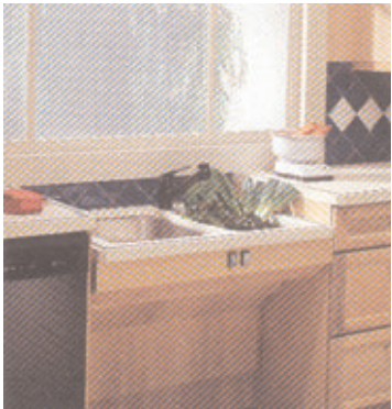
Adjustable sink height aids use by the disabled (courtesy, SWA).
