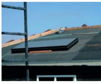
Photovoltaic roof panels are installed on a home built by Shea Homes in San Diego to increase the home's energy efficiency.
