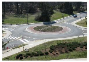
Modern roundabout used to increase throughput (compared to signals) and lowers speeds overall. Photo source: Andrew Bossi
