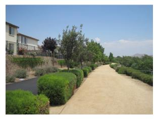
This trail made of decomposed granite allows rainwater to flow through, preventing flooding, while providing a solid surface for walking and biking. Photo source: Mike Singleton
