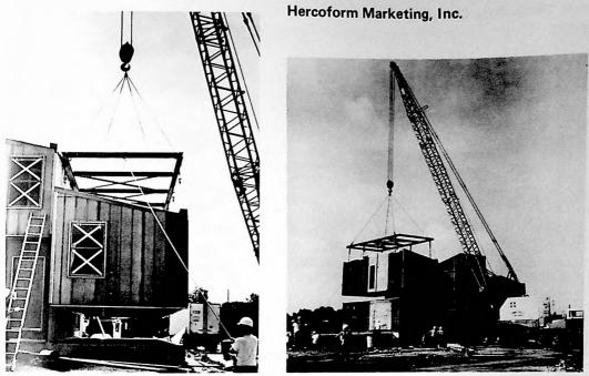
LONG BOOM CRANE USED BY HERCOFORM PERMITS PLACEMENT OF MODULAR CLUSTER FROM ONE LOCATION.
