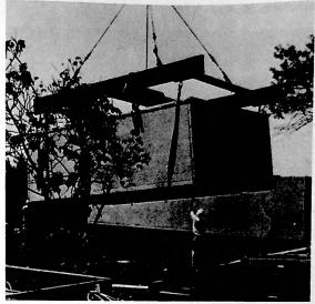
LIFTING FRAME WITH NYLON STRAPS
