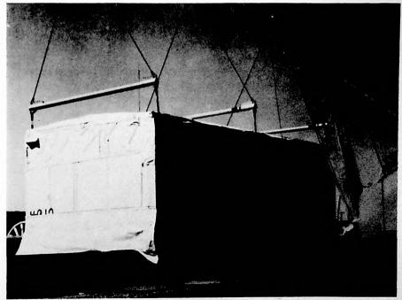
LIFTING FRAME WITH NYLON STRAPS
