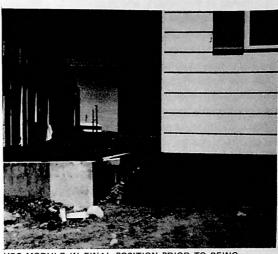
HBC MODULE IN FINAL POSITION PRIOR TO BEING TRANSVERSELY SHIFTED ONTO FOUNDATION. NOTE SLIDE RAILS BETWEEN FOUNDATION AND TRANSPORTER DECK.
