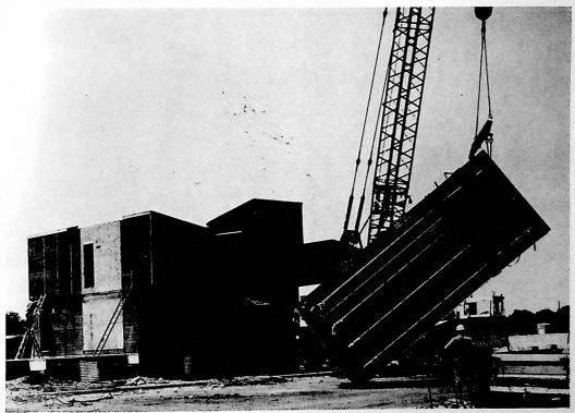
"TILT-UP" TYPE ERECTION OF HERCULES TOWER MODULE
