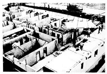
CEILING/FLOOR SLABS BEING PLACED ON WALL PANELS
