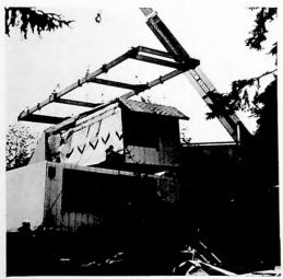
GUIDE ROPES ASSIST IN PLACING MODULES.
