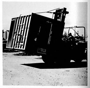
ALCOA'S MECHANICAL CORE MODULE BEING SHIFTED IN STORAGE YARD
