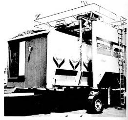
LEVITT STRADDLE CARRIER LOADING MODULE ONTO RAILCAR
