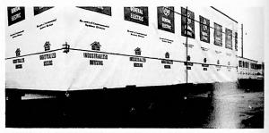
ORIGINAL PACKAGING THAT FAILED DURING FIRST RAIL SHIPMENT TO MEMPHIS AND WAS LATER REPLACED WITH CROSS-LAMINATED HIGH-DENSITY POLYETHELENE
