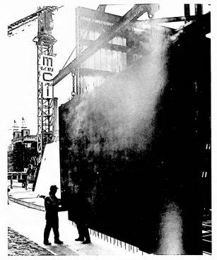
FLOOR PANEL BEING MOVED TO CURING AREA
