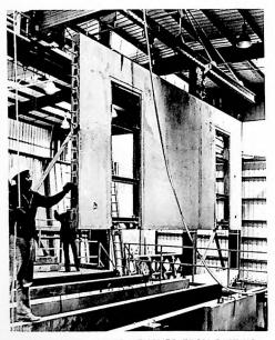
WALL PANEL BEING REMOVED FROM CASTING MOLD
