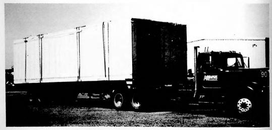
MATERIAL SYSTEMS CORP. MODULE SECURED TO TRANSPORTER WITH DACRON STRAPS
