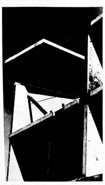
PRE-CAST CONCRETE CEILING/FLOOR PANEL IS LOWERED INTO POSITION.
