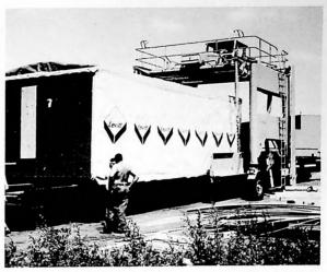
LEVITT PACKAGED MODULE BEING LOADED ON RAIL-CAR
