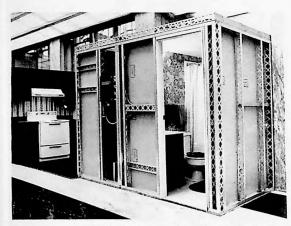
BATHROOM/KITCHEN MODULE UTILIZING INCOMBUSTIBLE ALCOA ALUMIFRAME
