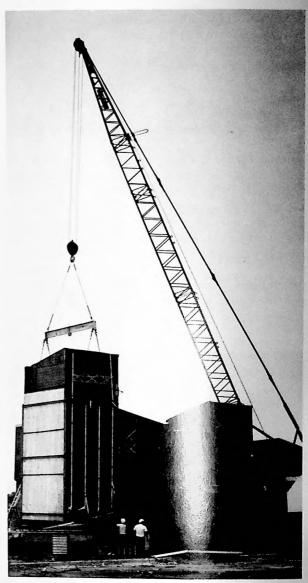
LOWERING "TILT UP" MODULE ON FOUNDATION-HERCULES
