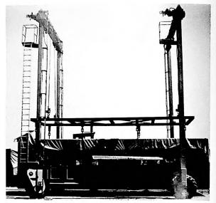
HIGH-LIFT CARRIER POSITIONS HERCOFORM MODULE
