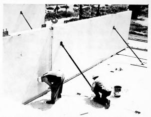
WALL-BRACING USED DURING ASSEMBLY OF DESCON'S UNITS
