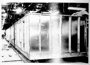
MODULE ASSEMBLY USING METAL STUDS
