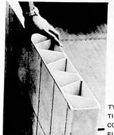
TYPICAL WALL CONSTRUC-TION SHOWING CORRUGATED CORE AND SURFACE ELEMENTS
