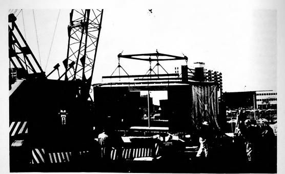
LIFTING FRAME BEING USED TO ERECT MODULES
