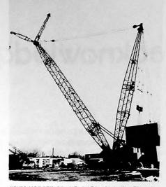
"SKY HORSE" CRANE, USED BY SHELLEY, TO HOIST AND POSITION CONCRETE MODULES AT JERSEY CITY.
