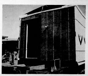
LEVITT'S RIGID SECUREMENT SYSTEM. NOTE 8" X 8" TRANSVERSE PREFORMED ANGLE IRONS AT MODULE'S BASE
