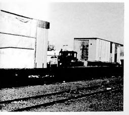
SECUREMENT OF BOISE'S MODULE TO LOW-HEIGHT RAIL CAR
