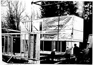
LIFTING AND PLACEMENT OF ALCOA'S MECHANICAL CORE AND ALUMINUM FRAMED WALL SYSTEM. NOTE THAT PROTECTIVE PACKAGING WAS RETAINED IN PLACE UNTIL AFTER CORES WERE ERECTED.
