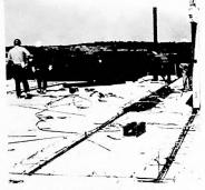
VIEW OF CAVITY AT JUNCTION OF WALL & FLOOR PANELS READY TO RECEIVE CONCRETE
