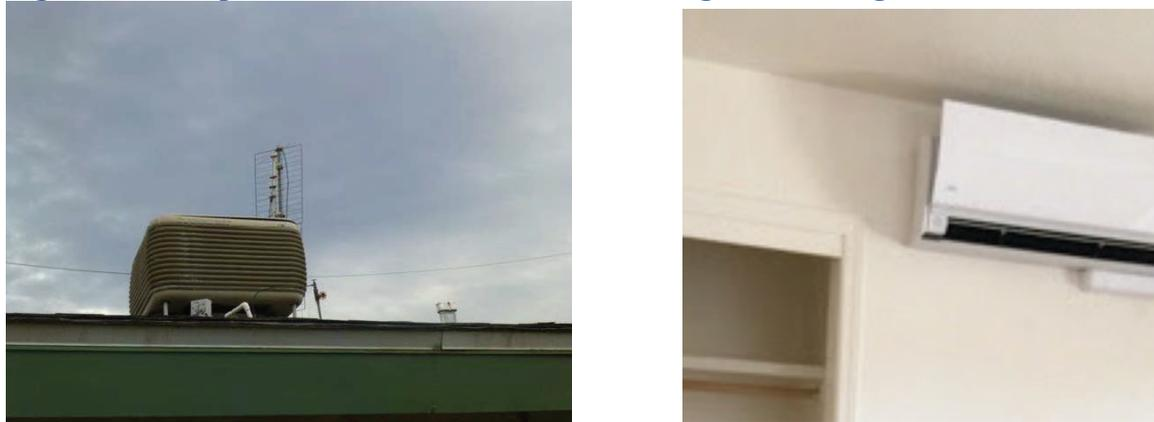
Swamp coolers (on the left, provided by FH) were replaced with the wall-mounted heating and cooling (mini-split) units, which were installed in each room.
