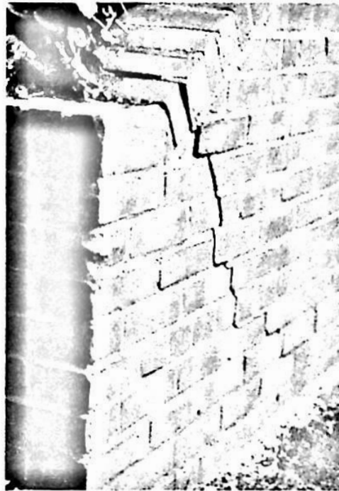
The outward movement of the upper part of this retaining wall can be halted only by structural reinforcement. Simply patching the crack will not solve the problem.
