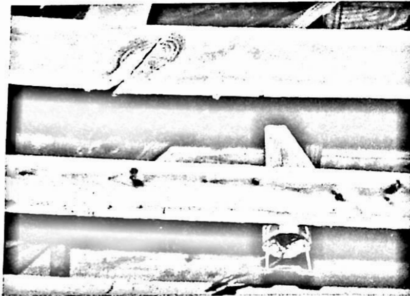
This split ceiling joist can be easily repaired by propping it back in place and bolting new structural pieces to each side.
