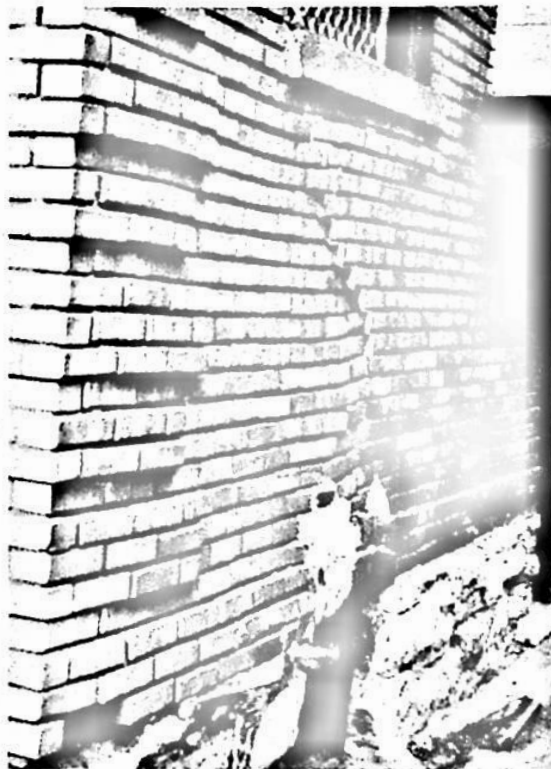
An extreme case of structural failure in a masonry wall due to foundation settlement. The wall and foundation must be completely rebuilt.
