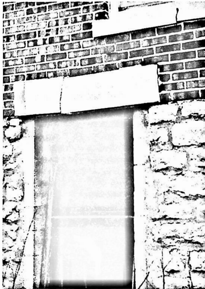
Failure of a concrete lintel and sill due to differential settlement of the building. Permanent repairs will be quite expensive. Note the makeshift shoring of the lintel.
