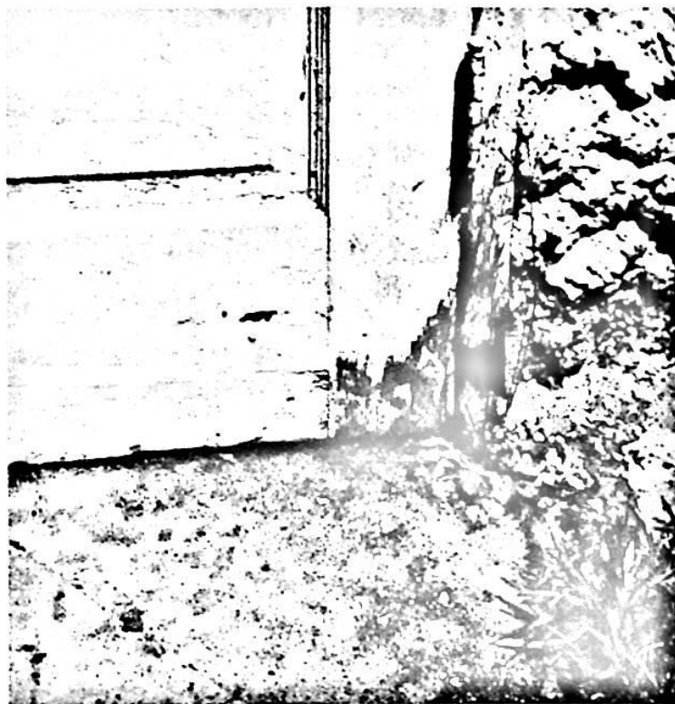
A common location of fungal and insect infestation is where wood door frames touch concrete or earth at grade.
