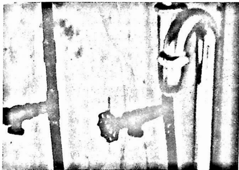
A S-trap that can cause self-siphonage and loss of the water seal. All such traps should be replaced.
