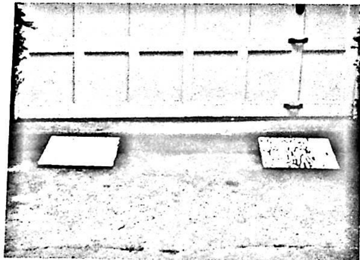
The concrete driveway is intact but has settled several inches. The only permanent solution is to replace this section.
