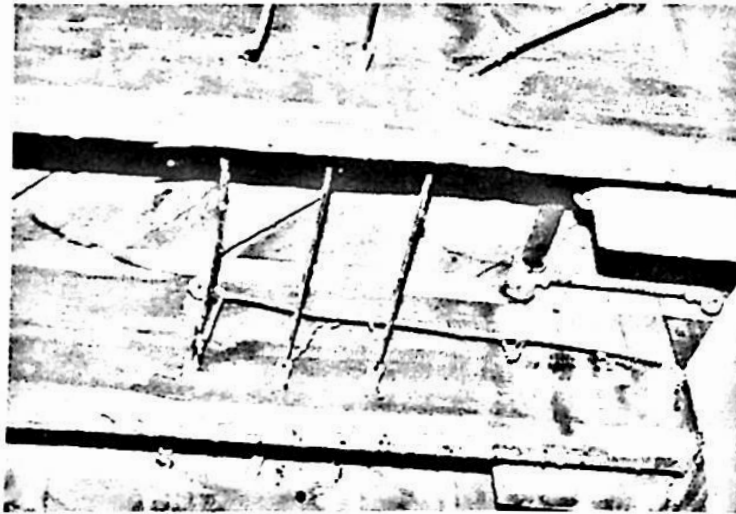
This knob and tube wiring is in good condition except for a piece of broken insulation (top of photograph), which should be taped.
