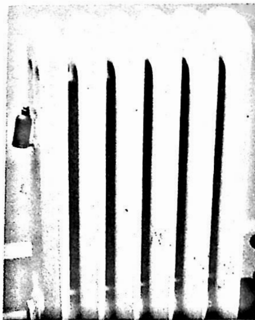
The hot water radiator on the left has a bleed valve at its top left corner. The steam radiator on the right has an air vent.
