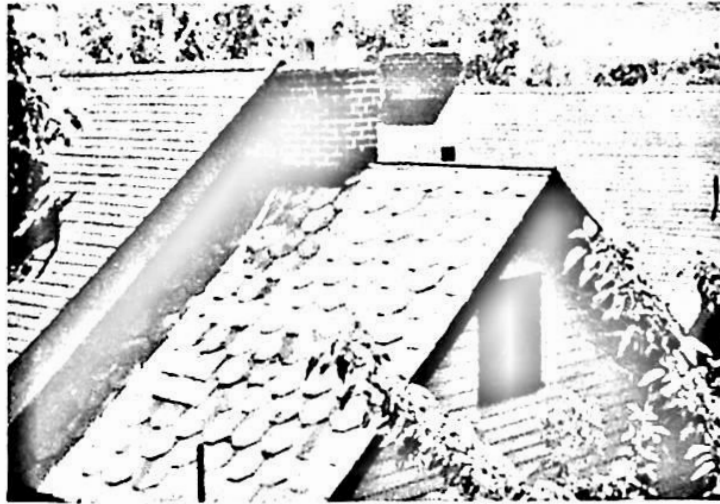
This slate roof should be carefully investigated since it has a makeshift repair. Other problems include the chimney, which is too low, and the vent pipe, which is too narrow.
