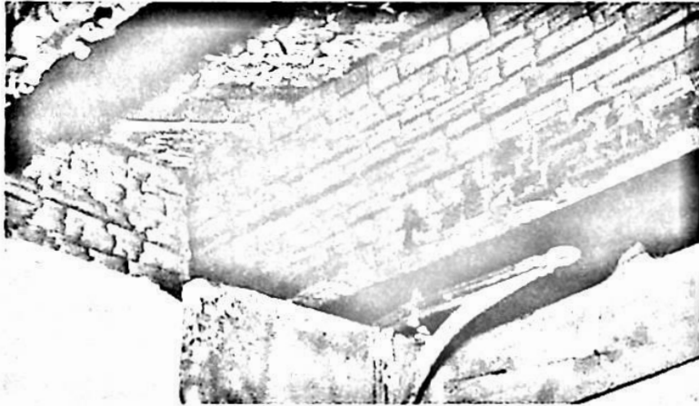
This fire damaged wood should be carefully probed to determine the extent of charring. In this case, the wood was replaced.
