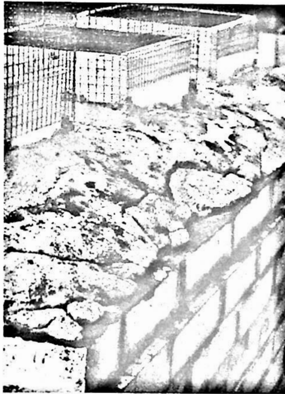
A deteriorated chimney cap. Mortar, rather than concrete, is often improperly used (as it was here) to cap the chimney. The masonry below will eventually deteriorate unless the cap is replaced.
